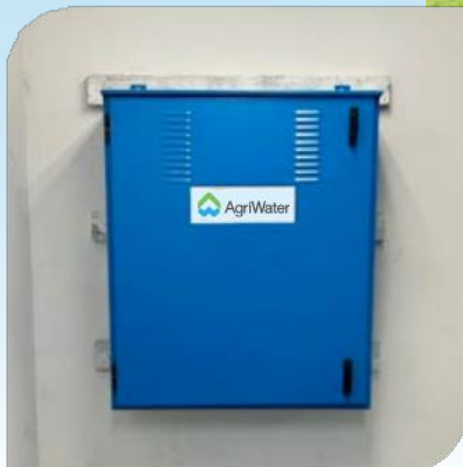
Agriwater Unit Install May, 2023
